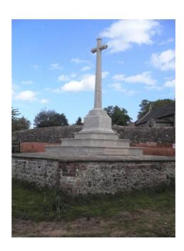
The bricks, including the coping stones, were sourced from a small brickyard in Aldeburgh, and the rebuilding including the flintwork was completed by Gray Developments in the summer of 2009.
